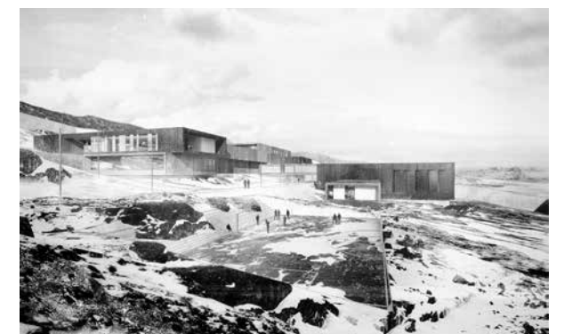
Schmidt Hammer Lassen recently designed the New Correctional Facility in Nuuk, Greenland, the first building of its kind in the country's capital.
